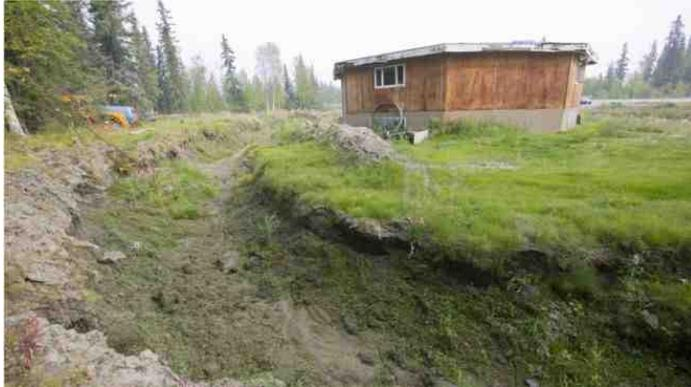
Houses like this one near Fairbanks have collapsed because of permafrost melt
