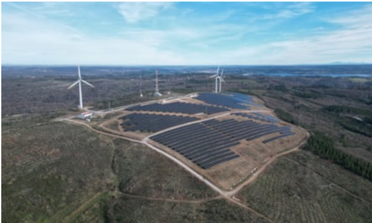
Hybrid power park with solar panels and wind turbines in Sabugal, Portugal. Photograph: Reuters
