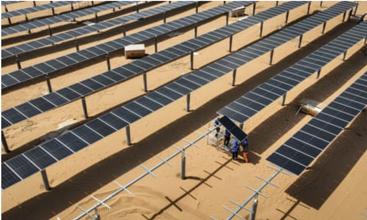
Solar panels under construction in Zhongwei, China. Photograph: AFP/Getty Images
