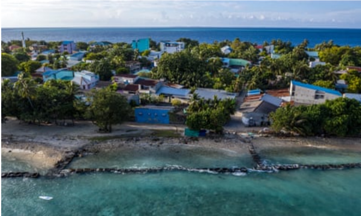
Concrete blocks are placed along the shoreline to try to prevent further coastal erosion, in Mahibadhoo, Maldives. Photograph: Carl Court/Getty Images
