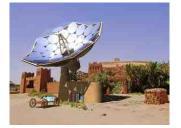
The 10-metre-high, sun-tracking dish has been designed to be transported in a single shipping container, so it can be delivered to any location. It is being developed by Airlight Energy of Biasca, Switzerland. As well as clean water and electricity, it can generate heat or, with the addition of a heat pump, provide refrigeration.
