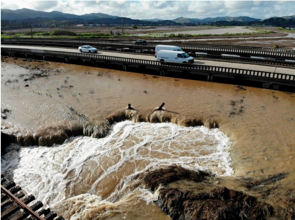
Water from recent heavy rainstorms breached a levee in Novato, Calif., on Feb. 14.
