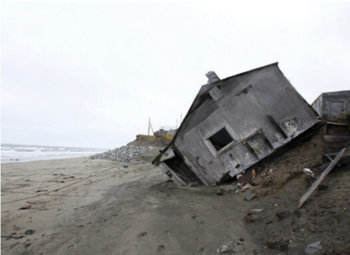
Beach erosion destroyed this home in Shishmaref, Alaska, shown in 2006; now the whole village must move because of sea level rise.
