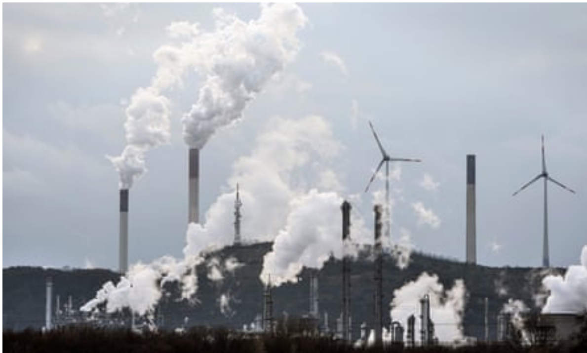
A BP refinery and a Uniper coal-fired power plant in Gelsenkirchen, Germany. Photograph: Martin Meissner/AP
