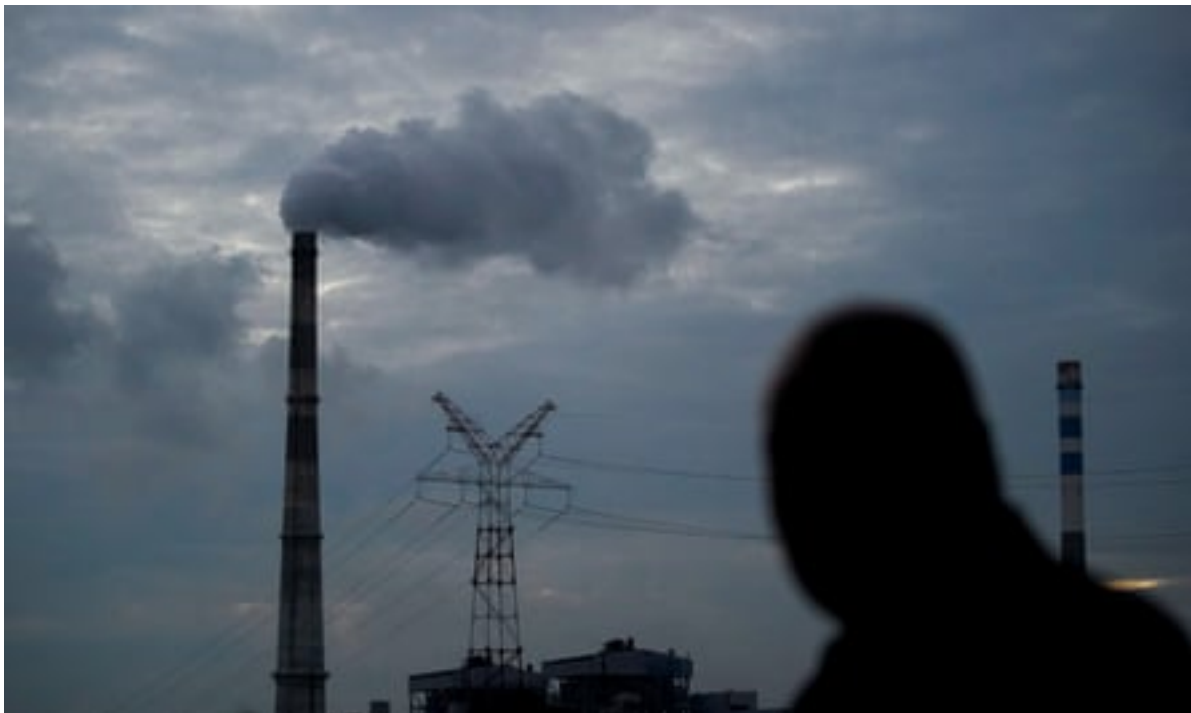
A coal-fired power plant in Shanghai. China approved more coal power in the first three months of 2023 than in the whole of 2021. Photograph: Aly Song/Reuters
