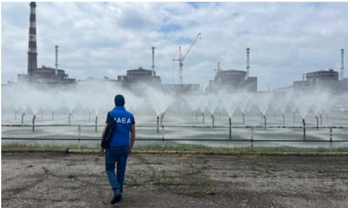
A member of the IAEA walking near the Zaporizhzhia plant during an official visit of IAEA director Raphael Grossi. Photograph: International Atomic Energy Agen/AFP/Getty Images
