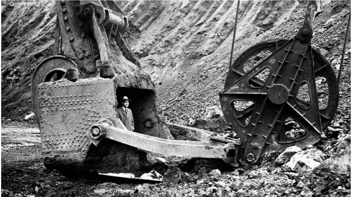
In 1929, a man stands inside a large stripper-type shovel at Fidelity coal mine, near DuQuoin, Illinois (Credit: Getty Images)
