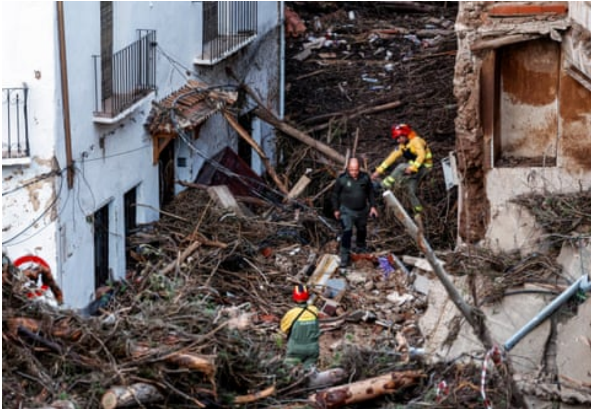
Members of emergency services work on a devastated street after flash floods in Letur, Spain. Photograph: Óscar del Pozo/AFP/Getty Images
